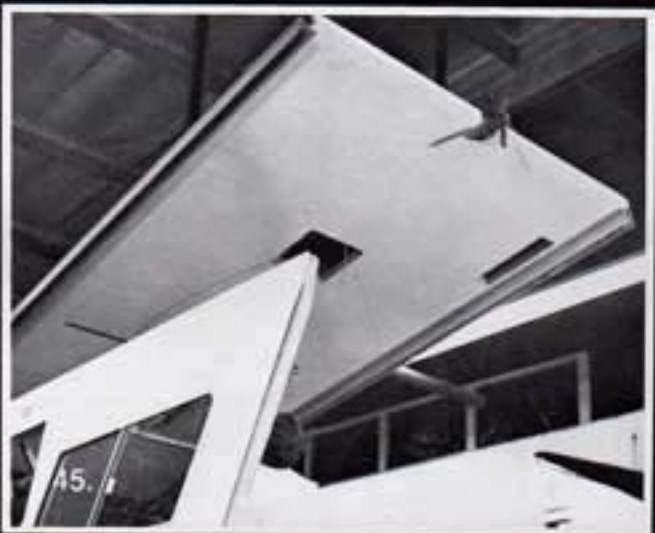
LOWERED INTO PLACE . . .
