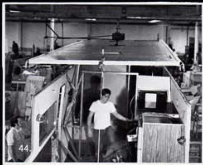
OVER THE WALL AND FRAMING STRUCTURE . . .
